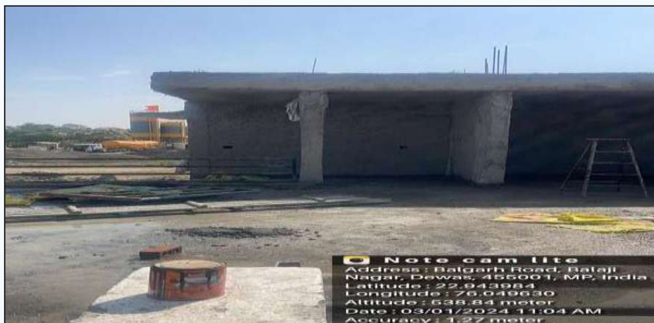
Image 24: Toilets under construction of the Government Model Higher Secondary School, Dewas, M.P. funded by BNP, Dewas, M.P.
